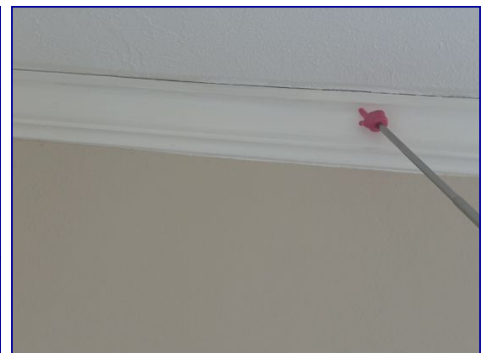
Crown Board separating
